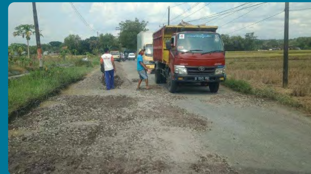
Maintenance and repairs of road used by local communities
